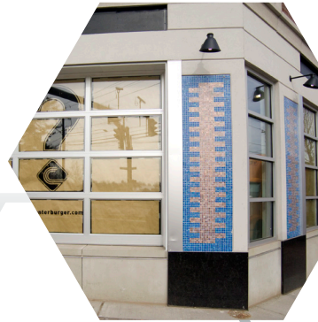
NATURAL STONE & GLASS MOSAIC INSTALLATION
